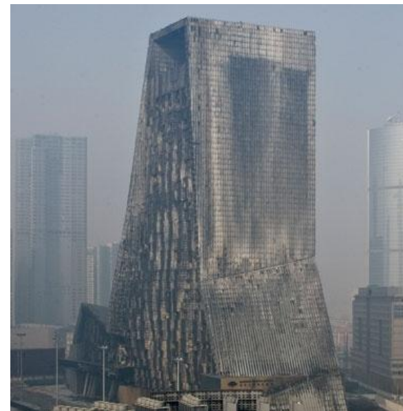
Mandarin Hotel Beijing Fire – February 2009 US$731m Damage
